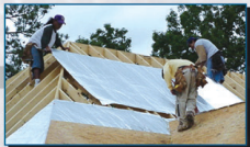
Beneath Roof Deck
